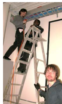
CCSF Students Installing BAVC Fiber
