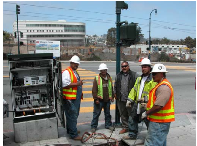
DTIS Crew Working on Fiber Install on Ocean Ave
