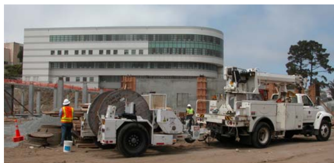
DTIS fiber installation coordinated with Wellness Center construction continued on page 3
